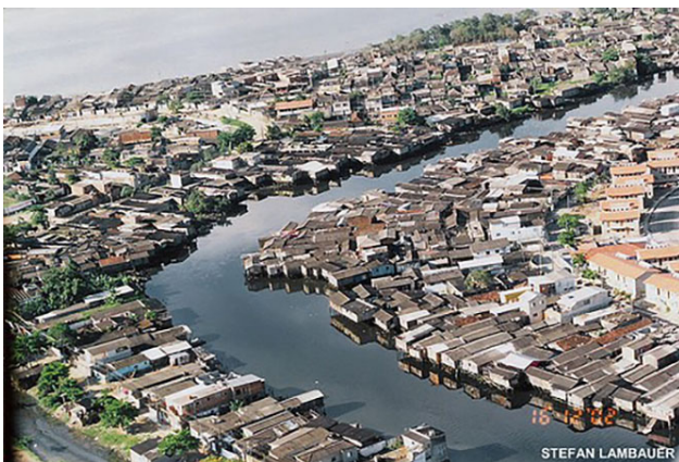
Figure 4 – Aerial view of Dique da Vila Gilda
