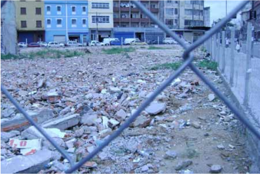
View of the area demolished on the corner of Protestantes and Mauá Streets (photo: Heitor Frúgoli Jr.).
